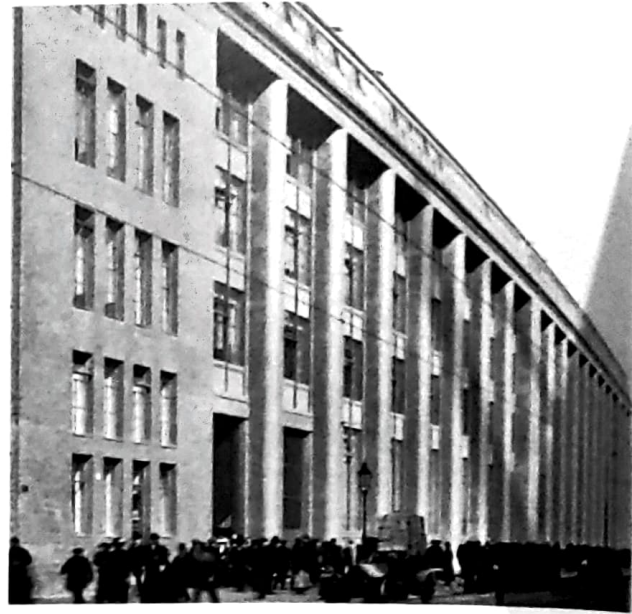
Factory for small engines
