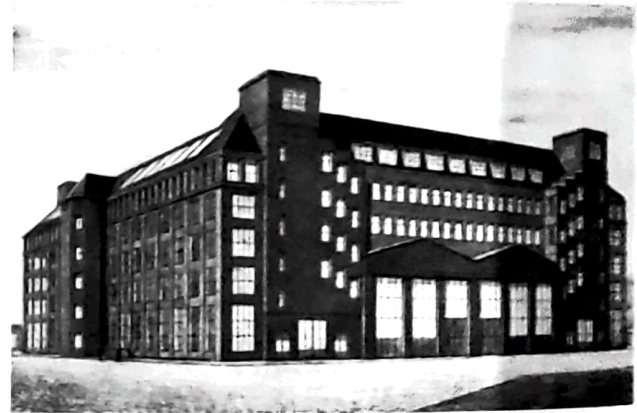
High-voltage transmission facility
